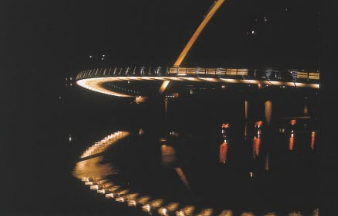
(previous spread) The Gateshead Metropolitan Borough Council is delighted with the entire project as it creates a successful visual impression at night, creating the iconic vision desired for the project. (left) Maximizing the opportunity for reflection, the underside of the deck is illuminated with custom luminaires. Positioned to reinforce the structure, the luminaires were designed with rotating and locking bracketry to allow maintenance from above the deck.
