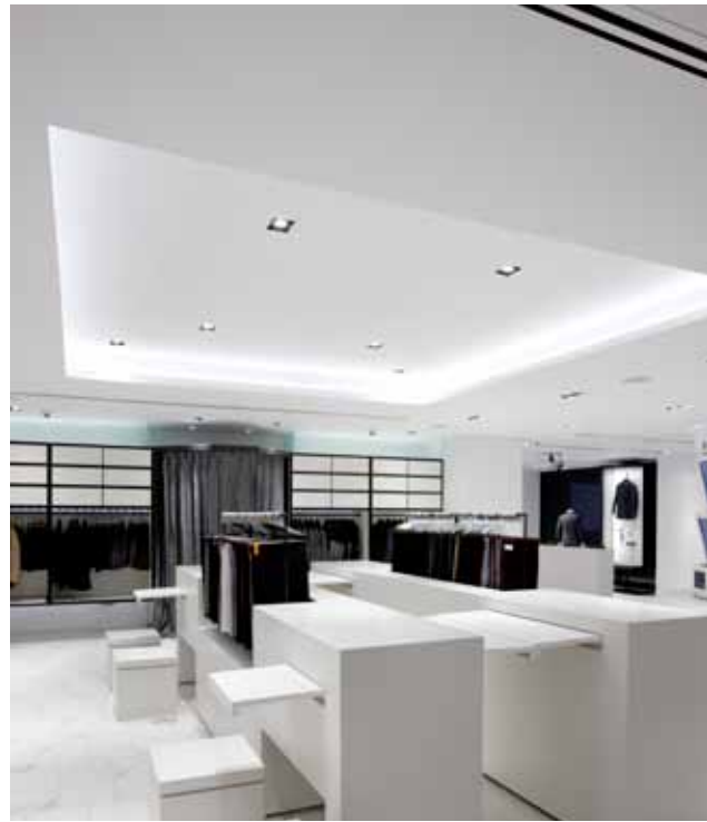
A square ceiling recess lined with warm-white LED cove frames the combination consulting station/fabric bar. Single metal halide track heads provide concentrated light for measuring tasks.
