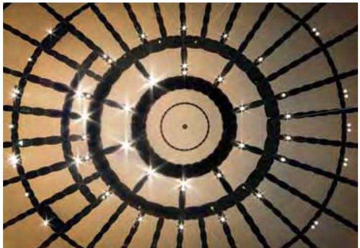
LED uplights illuminate the textured convex and concave acoustic walls (left). On the ceiling (right), clamp-mounted PAR 56 floodlights are mounted between fabric panels. Linked to a preset dimming system, the lights provide illumination for a range of events.
